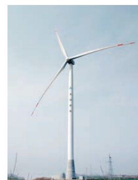
Hybrid (Steel-Concrete) Tower
