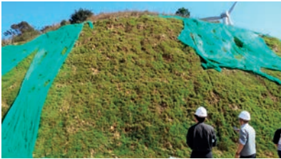
In the construction process of the Longgui Wind Farm, the Company took measures to restore the vegetation on the upper side slope of the excavation cross-section of the maintenance road in a timely fashion by planting grass on it using the "suspended net plus air-blast spraying" technique for sowing grass seeds.
