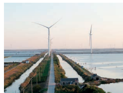
ⓘ Dafeng wind farm (50,000 kW) in Yancheng, Jiangsu
