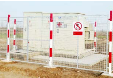
Putting up safety warning signs in the equipment area
