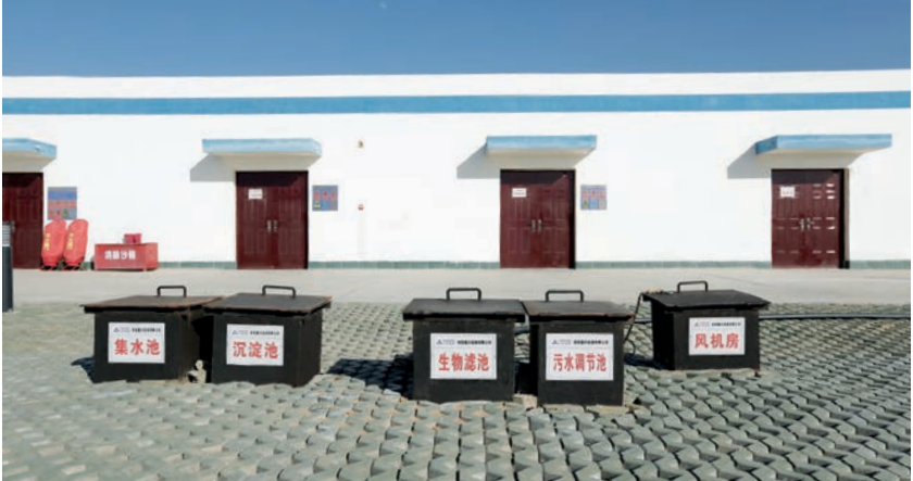
The waste water treatment facilities of wind farms
