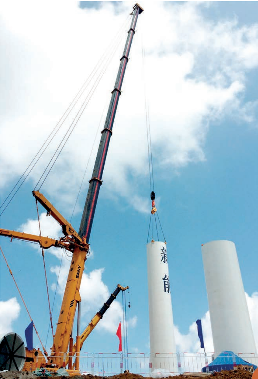
Ensuring safety of craning operations
